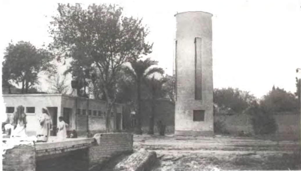
Water tower & washing places
