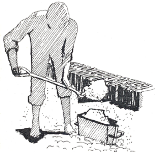
Fig. 4.25 The concrete can be compacted by hand in moulds (Ref. 20).
