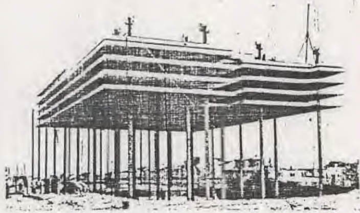
Lift-slab structure in the course of erection, USA
