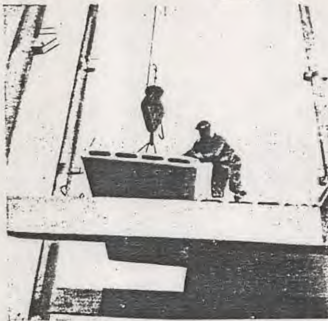
Erection of a building comprising tubular spun concrete columns, Bulgaria
