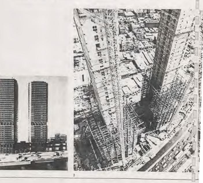
Bridge had to revert to the time-honouzed and traditional method of 'stick and winch', The majority of the steelwork has, however, been erected using our Potain cranes with the relp cf closed circuit television, bilingual banksmen and a very high degree of expertise by our expatriate H and H crane drivers.
